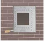
Screw the fixture on the wall by using 4 plugs and screws
