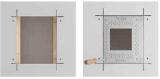
Cut a hole in the wall and install 2 wooden planks (dimensions: see technical data sheet)
