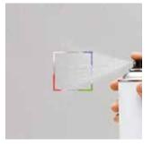
COAT\_SPRAY\_COMP Spray a matte water-based varnish on the switch to protect it and make it cleanable
